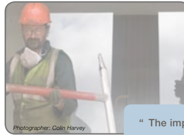
Contractor working on the National Gallery East Wing Renewal Project
